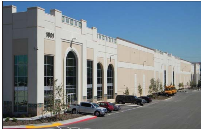
The front of our newest facility, Hunter Park, which opened a few months ago.
