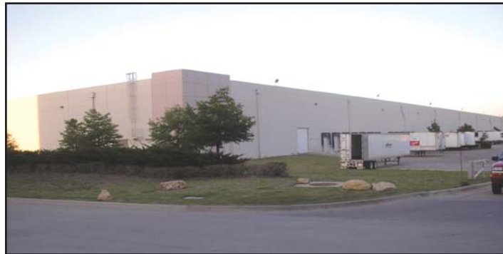
A view of the exterior of Building A in the three-building complex that comprises the Ft. Worth facility.
